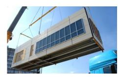
Offsite construction improves sustainability, worker safety, and quality by utilizing advanced design and materials, and innovative assembly techniques. It includes volumetric construction, which encompasses modular and pod building, prefabricated assemblies and panelized construction, where flat panels for walls, floors, roofs, and other building components are produced offsite.
