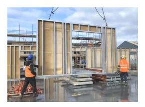
These panels are ideal for multi-story structures like hotels and multifamily buildings, as they can provide structural support with no or minimal iron or concrete columns. I-beams may be added for large spans or openings.
